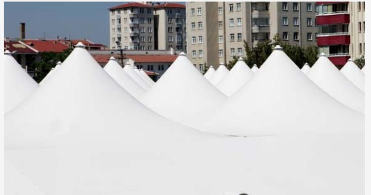
It is a strained system applied on four feet, with a conic shape and made of high quality PVC membrane textile. The main cage is steel construction and coated with special zinc. The system is designed with modular features and can be used to create endless areas.
